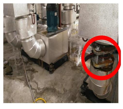
Example of a failed bellows in a LPHW system where hot water (85°C) at 1 bar was released suddenly across the plantroom floor.
