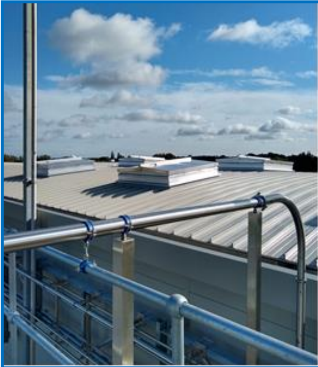
External view of roof hatches
