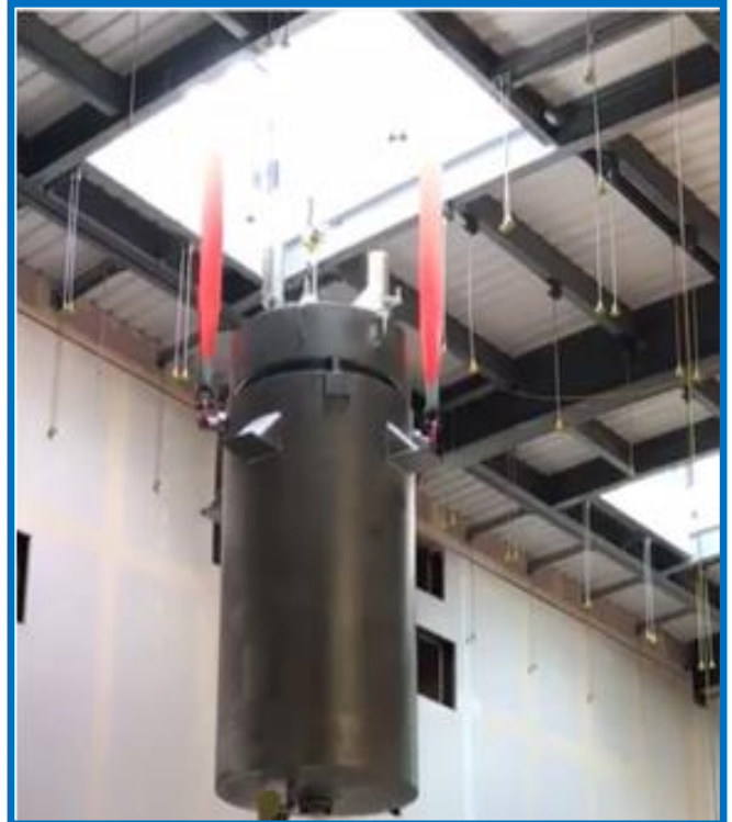
Vessel being lowered through hatch
