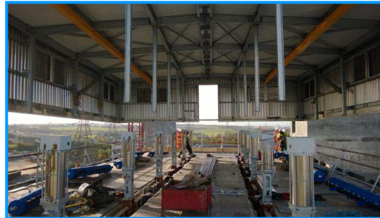
Module Being Lowered.
