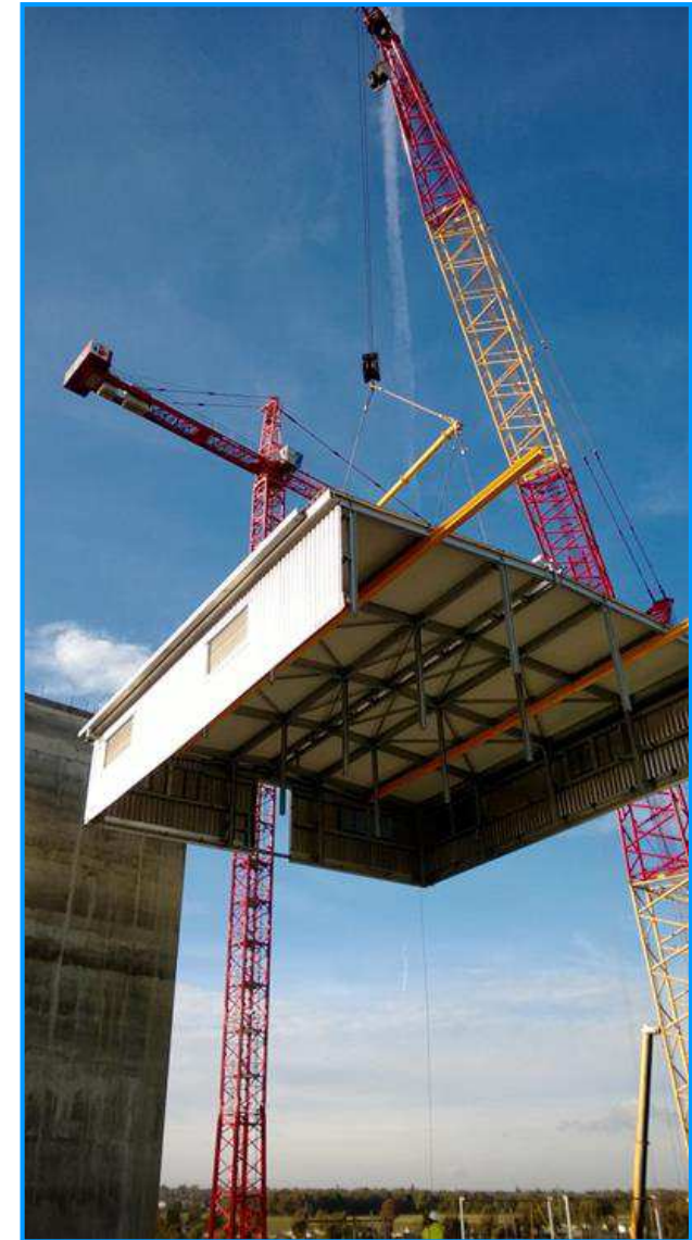
Module Being Lifted
