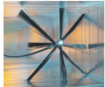
The machine can clean both rectangular and circular ductwork from 80mm diameter / square up to 900mm effectively. Re-sealable access panels (only 120mm diameter) can be cut into the existing ductwork up to 30m apart meaning access into the ceiling void / service risers of an existing building is limited. By using CCTV to inspect the ductwork before and after cleaning and to control the cleaning, where necessary, the entire process can be recorded for clients to keep to prove the cleanliness.
