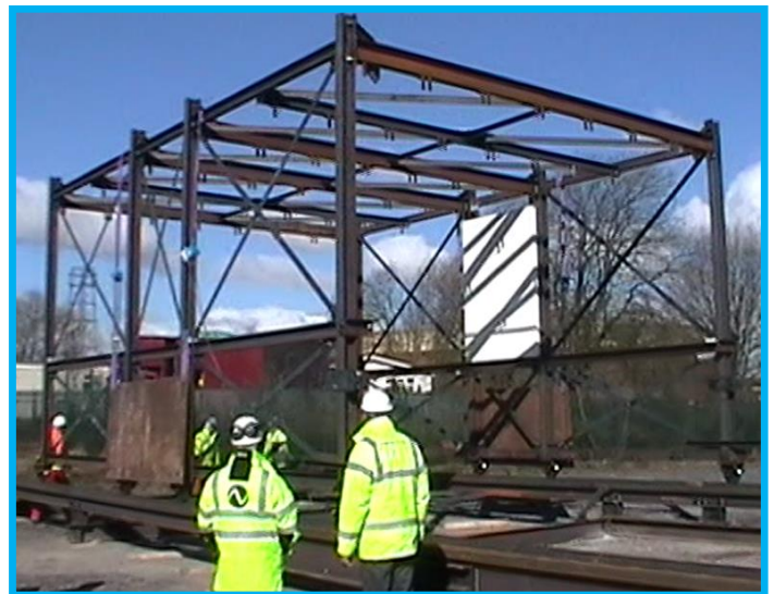
Final Structure – Before Cladding
