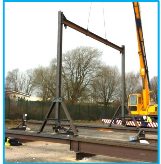
First Frame with Supports
