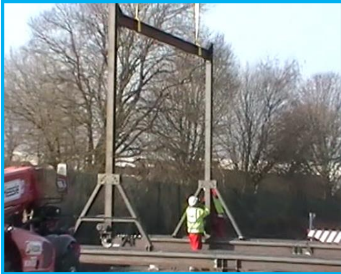
First Frame being erected
