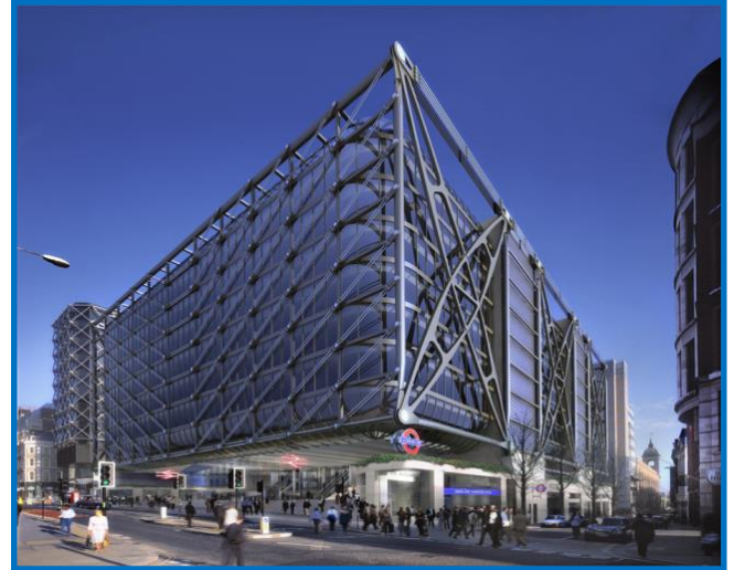
Cannon Place Bridge Structure
