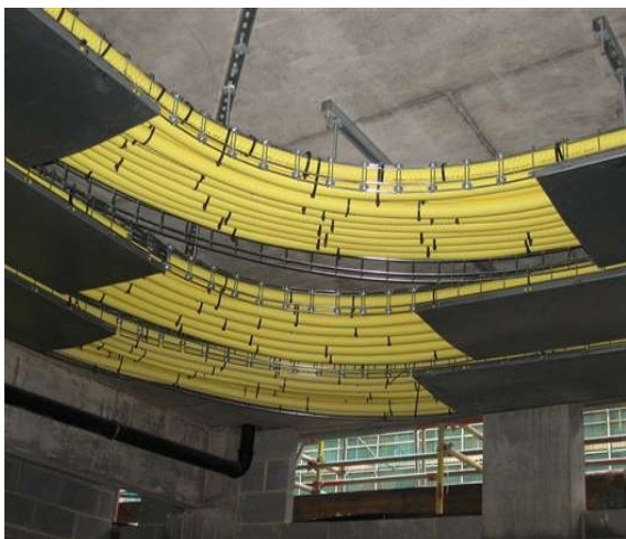
Tracpipe Installation
