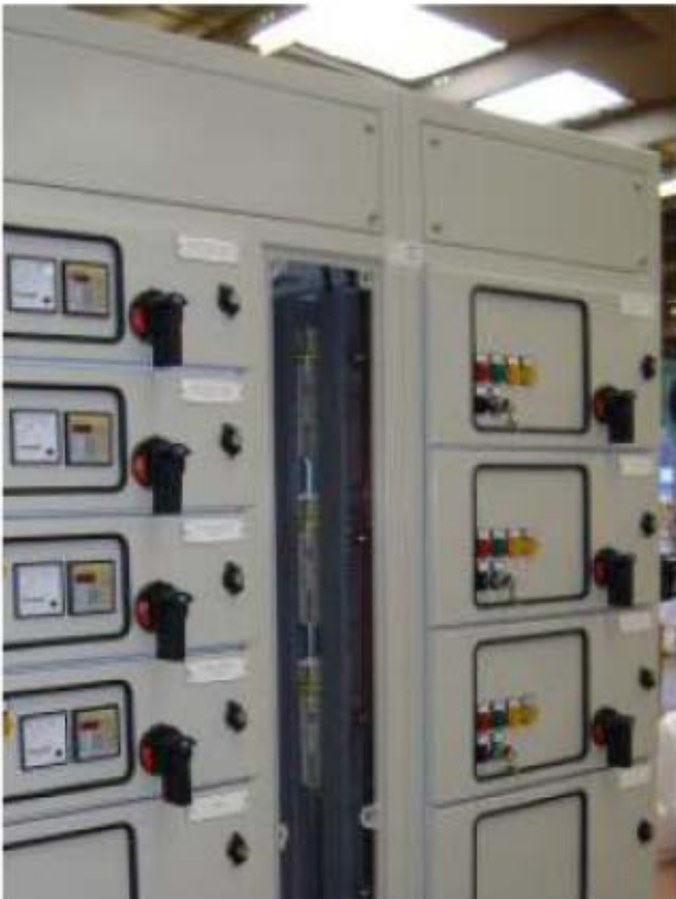
Left: Withdrawable MCC showing used and spare trays
