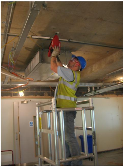
Fixing gas fired anchors to a concrete ceiling
