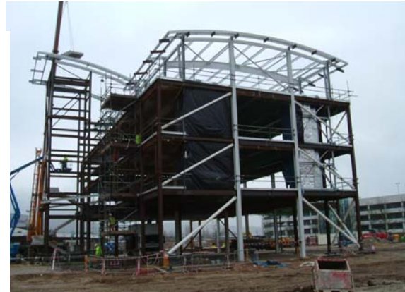
2 Gable Riser Modules.
