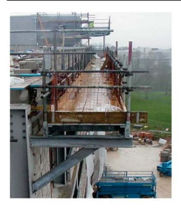
This project was designed with a stone parapet around the perimeter of the roof which would normally necessitate a full height scaffold from ground level (approximately 23m high)
