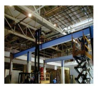
Two 4.6m x 4m roof construction accesses with hydraulically operated doors were provided through the existing beam and pot roof of the building to facilitate the safe removal of demolition material away from an occupied operational building and a congested and heavily trafficked area on the ground. These openings were programmed in to the construction activities and provided both a safe opening and closing mechanism and a quick method of weathering.
